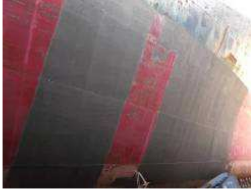
Blast cleaning (vertical bottom)
