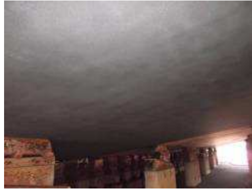
Blast cleaning (flat bottom)
