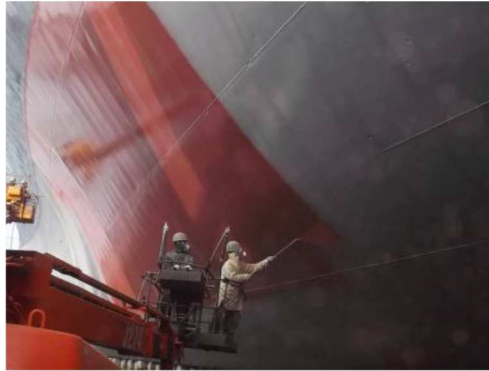
1st Application of A-LF-Sea
