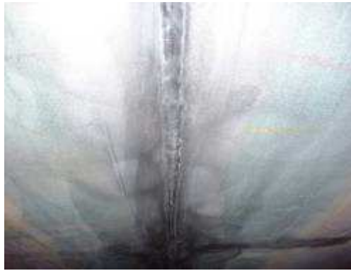
Surface preparation of erection joints (Power tool cleaning)
