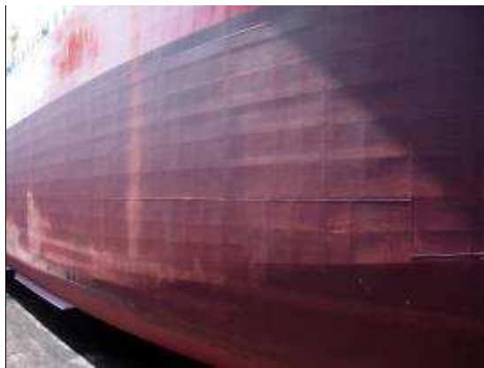
Removal of dirt - Power tool cleaning
