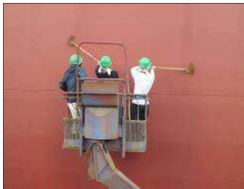
Dust removal by broom
