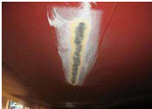
Surface preparation for burnt part
