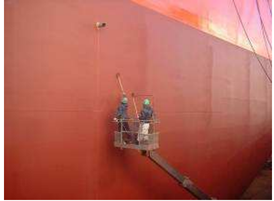
Removal of paint dust before final coating
