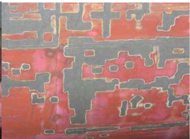
Square blast cleaning
