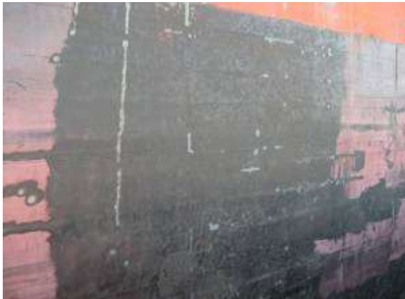
Loose paint film (Partial blast cleaning)
