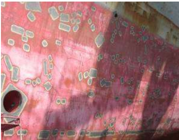
Square blast cleaning
