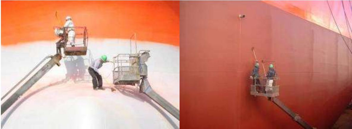
Removal of paint dust of finish coating adhered on bulbous bow
