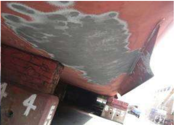
Rust scale or blistering (Partial blast cleaning)
